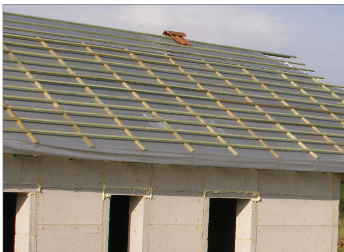
Battens, underlayment on roof structure
